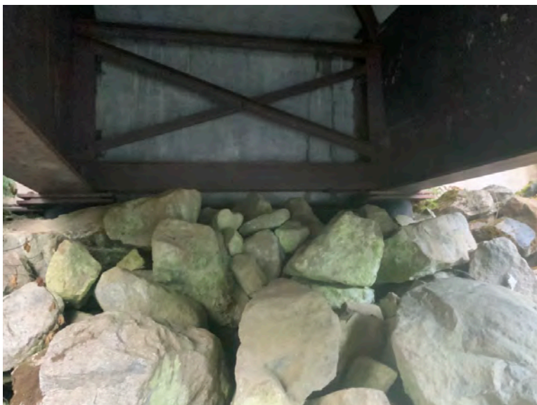
Right Bank Abutment when facing downstream
