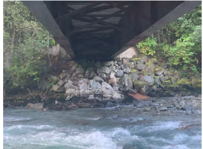
Right Bank Abutment when facing downstream
