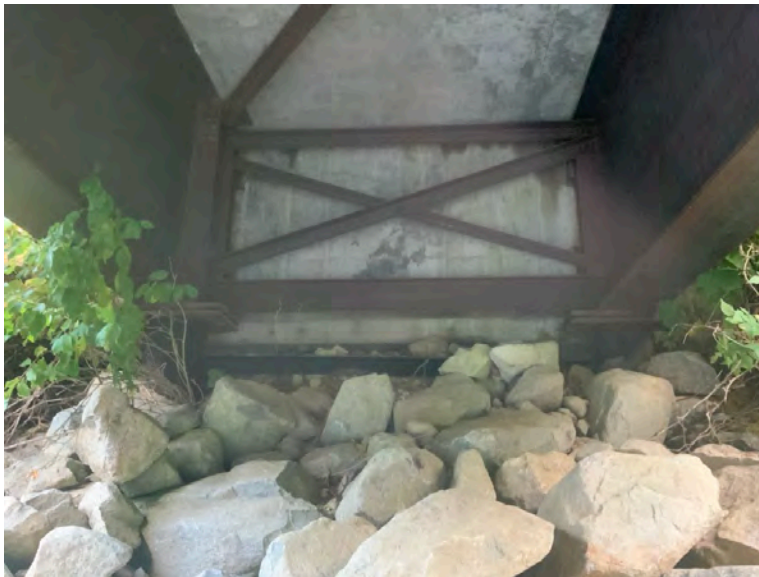
Left Bank Abutment when facing downstream
