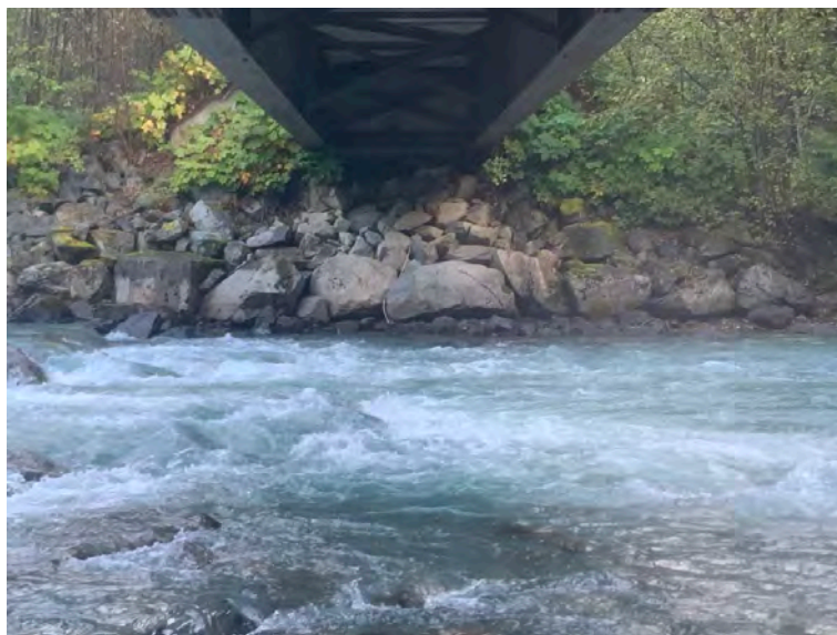
Left Bank Abutment when facing downstream
