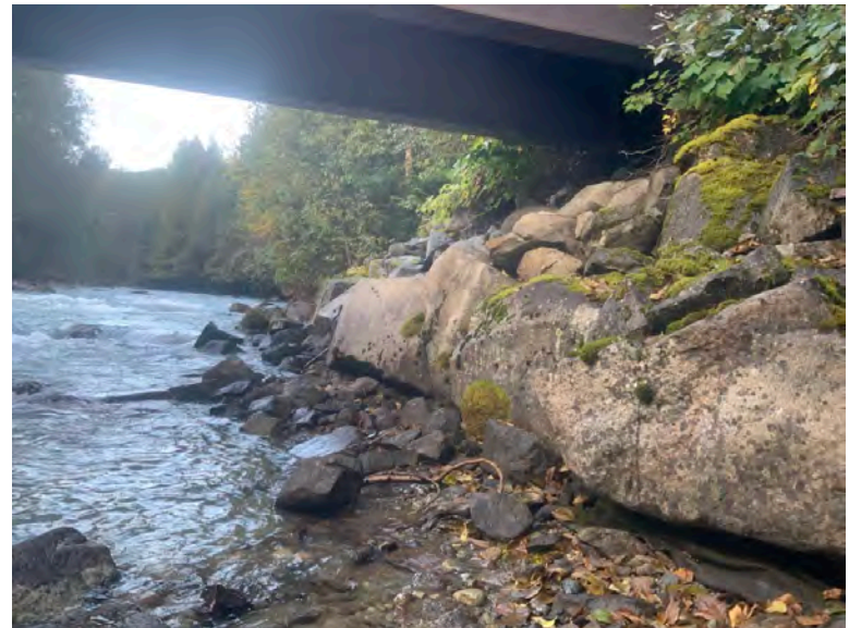
Left Bank Abutment when facing downstream
