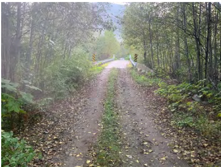
Approach from Right Bank when facing downstream
